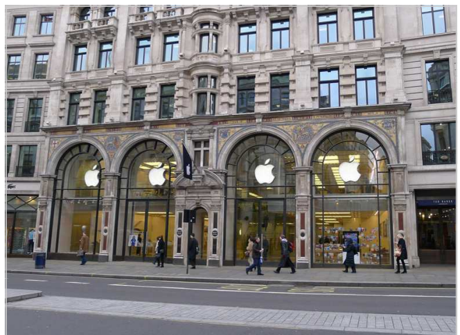
Above: By considering the architectural style of the building and utilising more appropriate materials and colour palettes even more modern designs can often be successfully integrated into the overall building façade.
